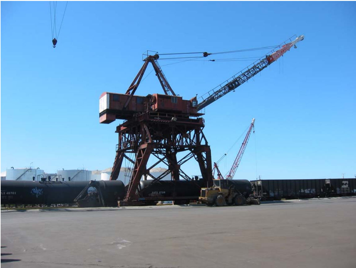
The historic Whirley Crane weighs nearly 500 tons and will be moved via barge and a 500-ton crane from Manson Construction used for bridge construction and retrofit work
